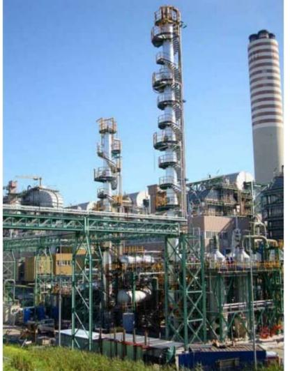
Approx 100 tpd CO<sub>2</sub> pilot on coal flue gas
